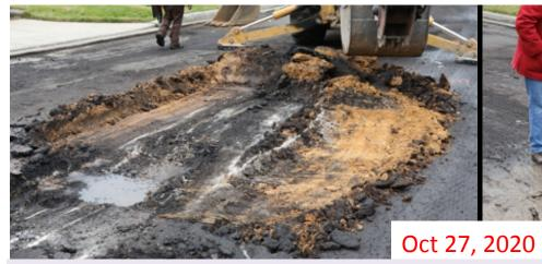
Oct 27: DDOT paving contractor's exploratory excavation uncovered a 4-foot-deep sink hole (*see shovel above*) and unstoppable water flow. Paving crew called DC Water, who arrived on the scene on <u>Oct 29</u> and tested the water.
