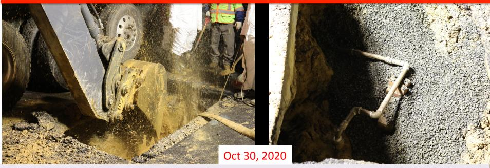
Oct 30, 2020: DC Water contractor performed repair to ruptured 1-1/2 inch service feeding 1762 Redwood Ter.
